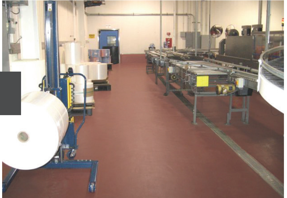
Stonclad UT replaced an unsafe, failing epoxy floor in Cold Springs Brewery's batching rooms.
