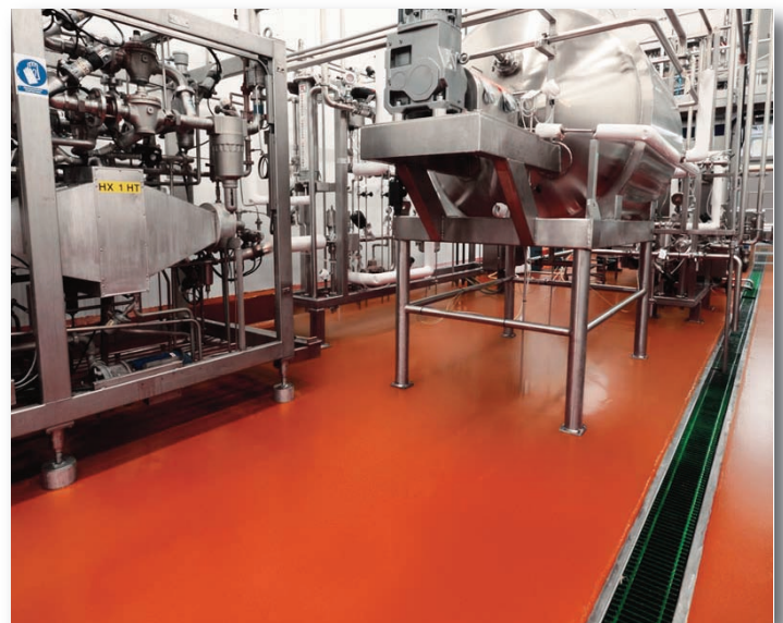
Seamless floors help prevent containment issues
