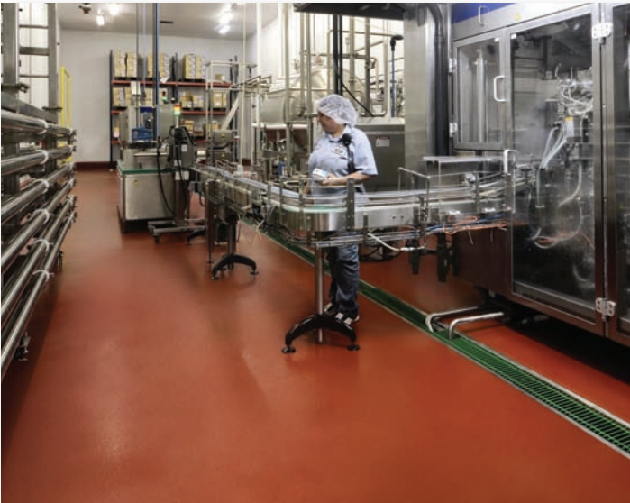
Stonhard installed Stonclad UT in the production area of Wright Foods. The floor is easy to clean and slip resistant.
